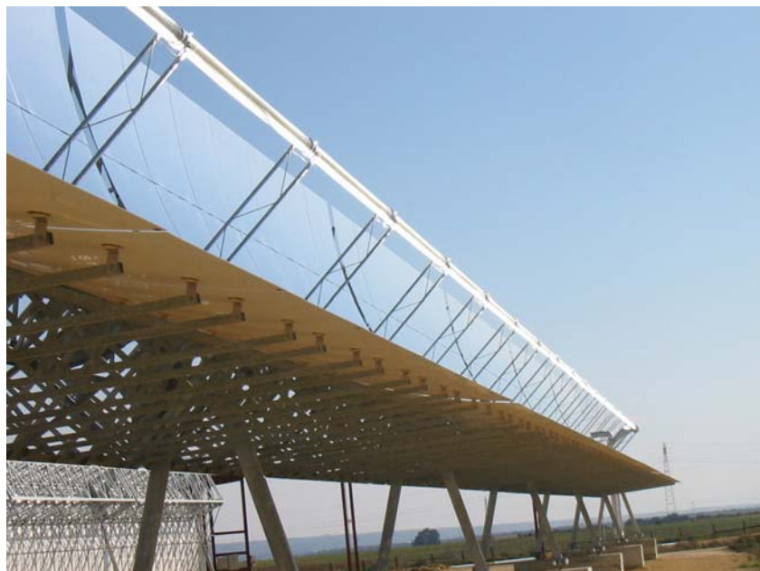
Figure 15: Abengoa Solar Trough
