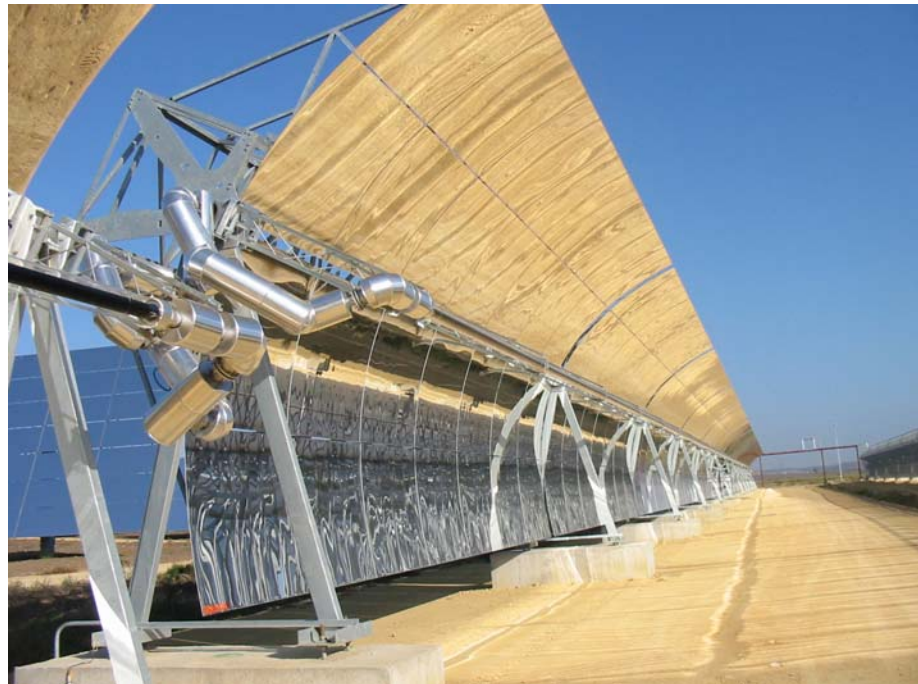
Figure 14: Solnova 1 under construction
