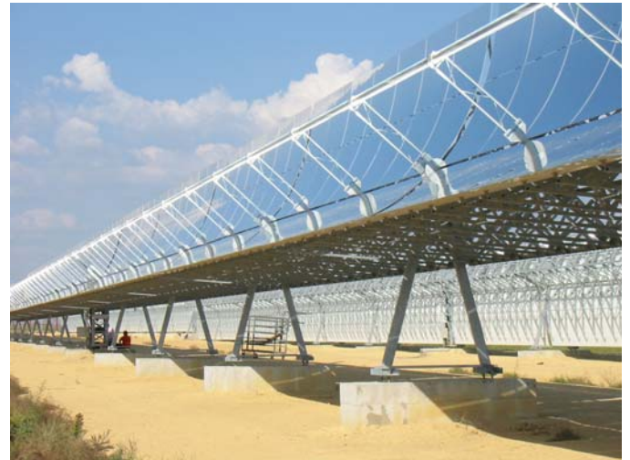
Figure 1: Solar Thermal Technology
