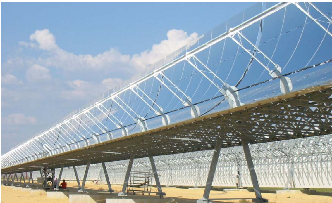
Figure 11: Abengoa Solar' Trough
